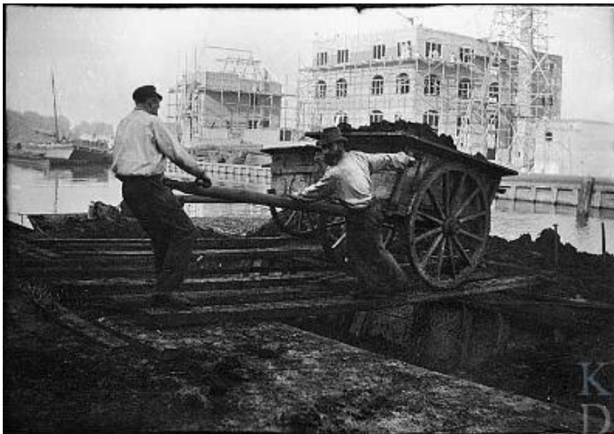
Barrow-men with sand carts on the Jacob van Lennepkade; in the background the office and factory buildings of the Fijnhout sawmill factory (under construction), 1900-1901. RKD Collection
